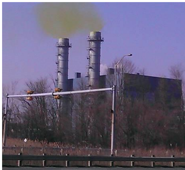
Figure 1: Yellow plume from on-site power generation
